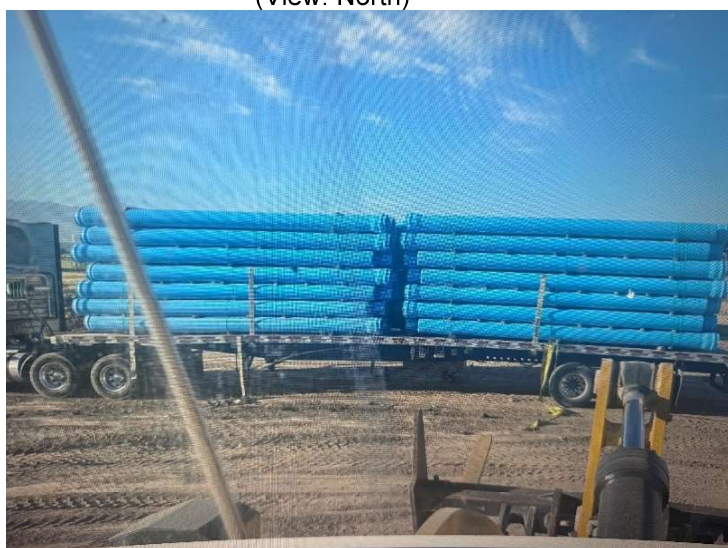
Water Pipe Delivery (View: N/A)
