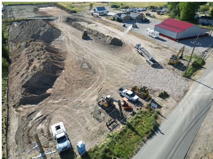
Construction Access (View: Southeast)
