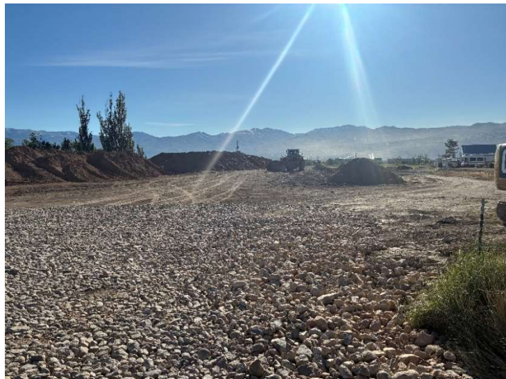
Construction Access (View: Northeast)
