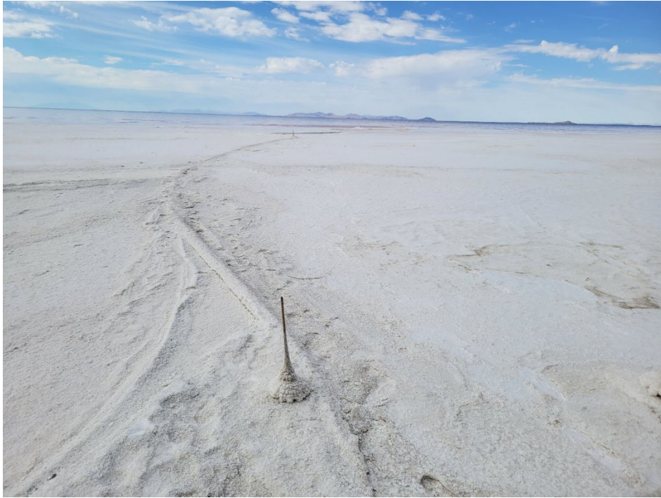
Centerline staking, looking West.
