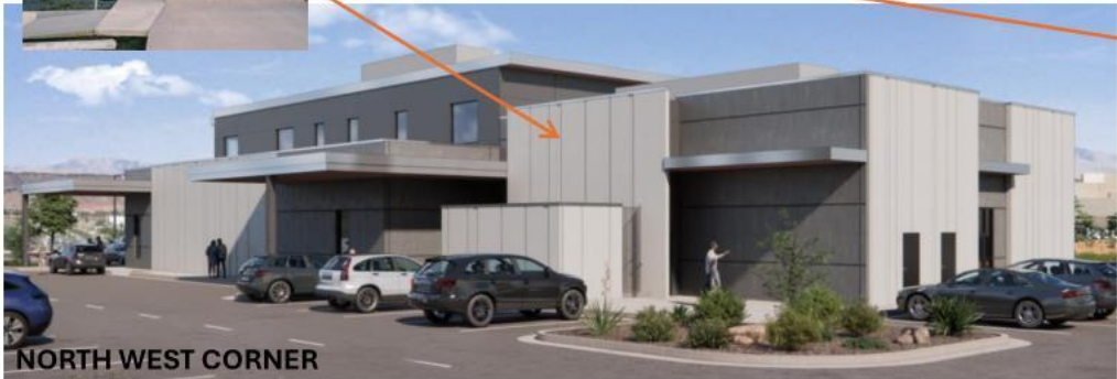
NORTH WEST CORNER
