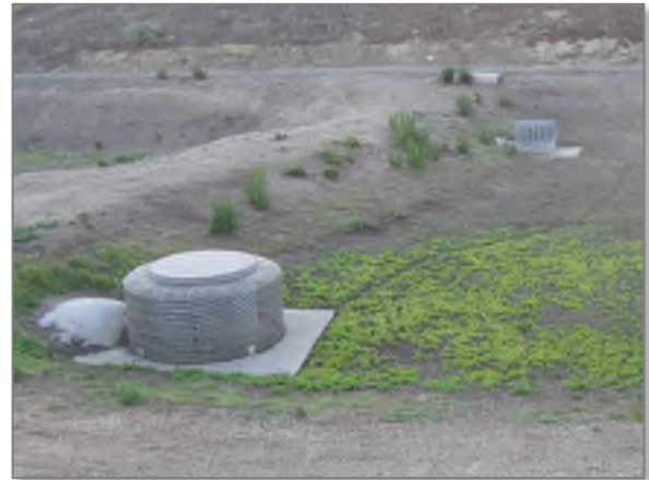
Figure 4: Multi-stage overflow outlet with trash screen
