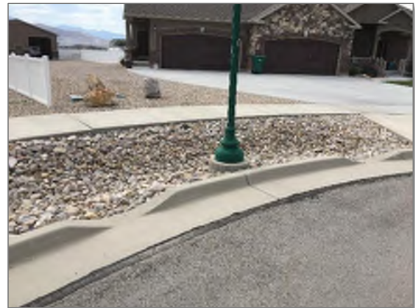
Figure 8: Curb cuts to a rock lined swale.
