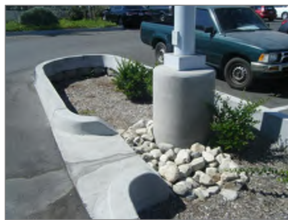
Figure 3: Retrofitted island curb within parking lot
