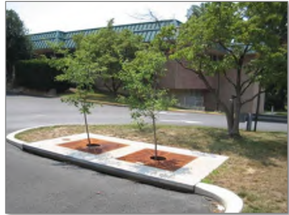
Figure 13: Proprietary tree box filter
