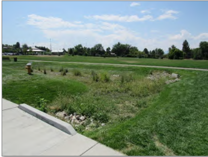
Figure 20: Bioretention area at Mountview Park.
