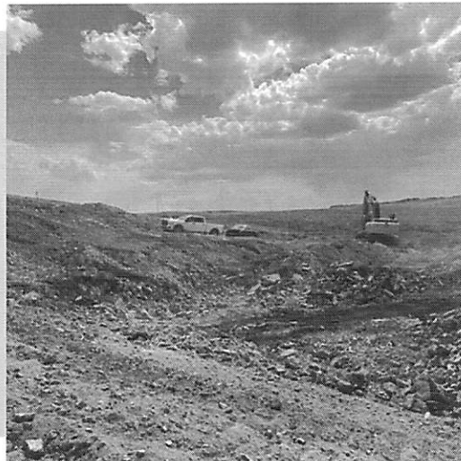
New Road Construction, Carbon Co. Wy
