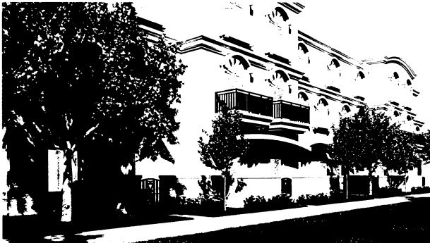
BUILDING A1, & A2 FIRST FLOOR RESIDENTIAL RENOVATION - EAST TO WEST VIEW
