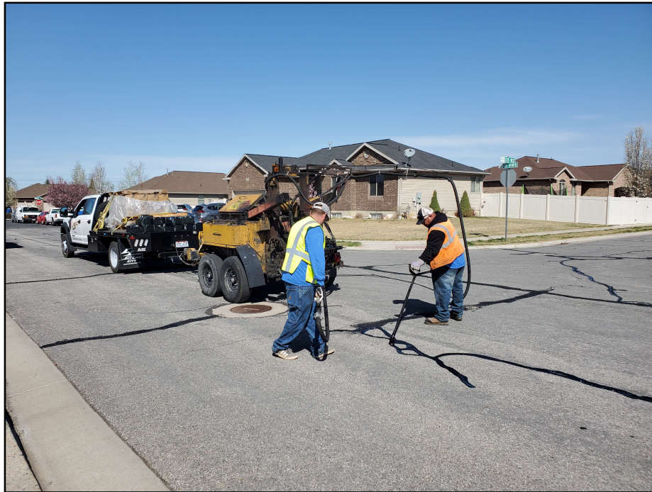
Figure 9. Crack Seal Treatment.
