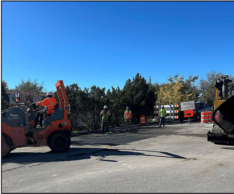
Figure 12. Asphalt Patching
