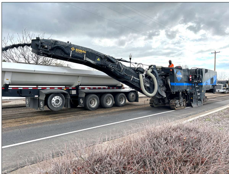
Figure 11. Asphalt Milling.
