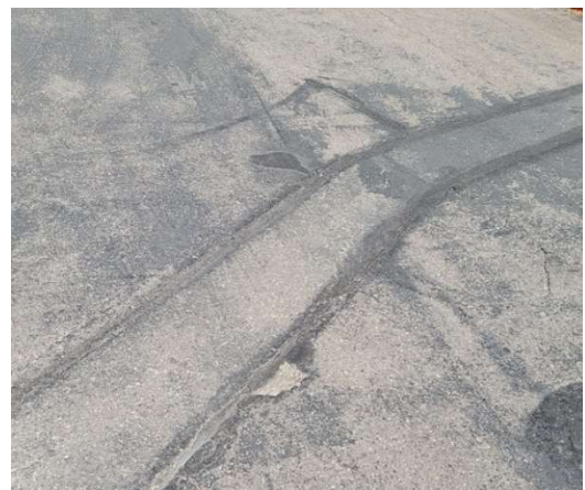
Figure 5 EXAMPLE OF PATCHING ON PAVEMENT
