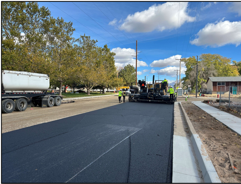
Figure 13. Asphalt Replacement.
