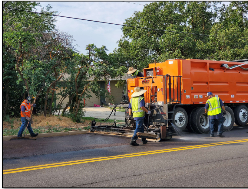
Figure 10. Slurry Seal Treatment.
