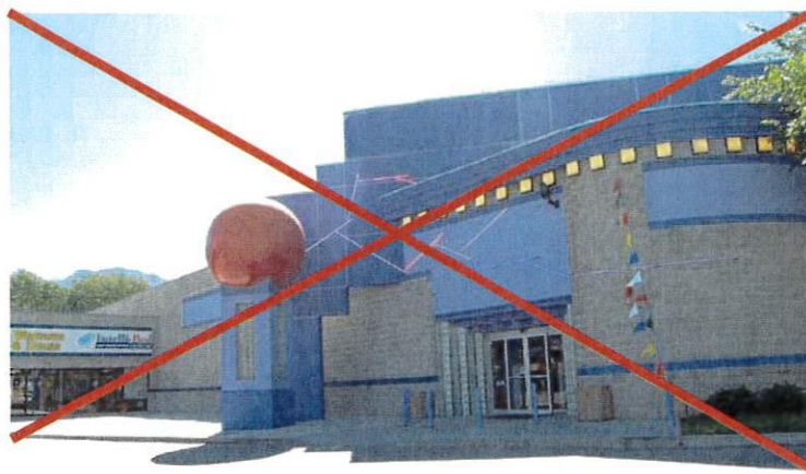
Not Permitted: bright colors and creative architecture overpower the building form and clash with architecture and theming of neighboring buildings and community
