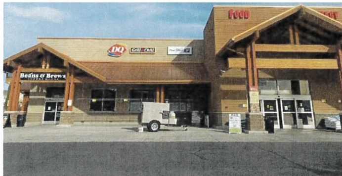
Required: Clearly identifiable covered entry
