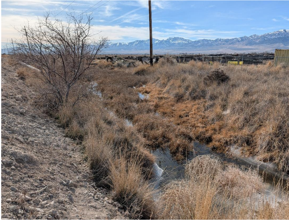
Figure 5-Surface water prior to culvert at Higley Road.
