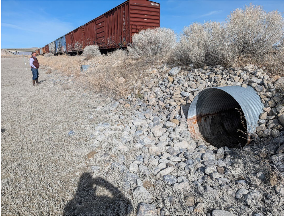
Figure 1-Location of proposed Outfall 001, looking north.
