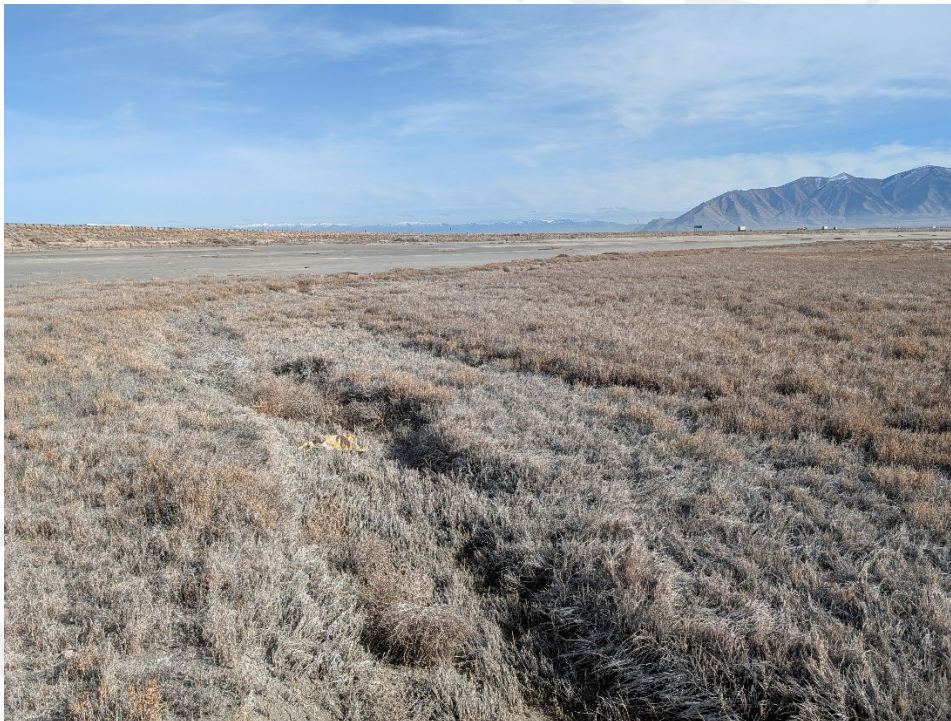
Figure 4-Downstream of railroad culvert at Outfall 001.
