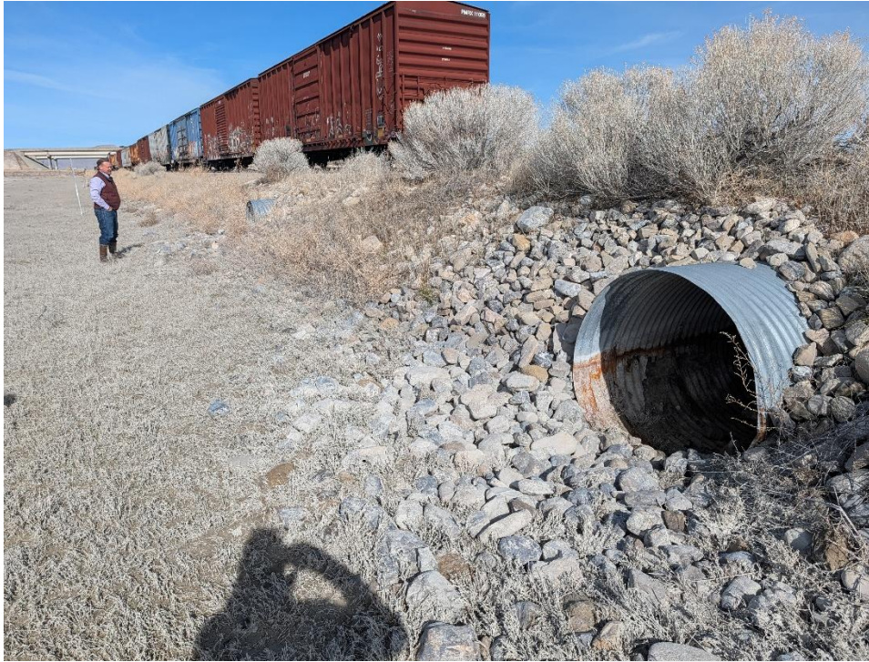
Figure 1-Location of proposed Outfall 001, looking north.
