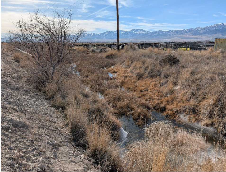
Figure 5-Surface water prior to culvert at Higley Road.
