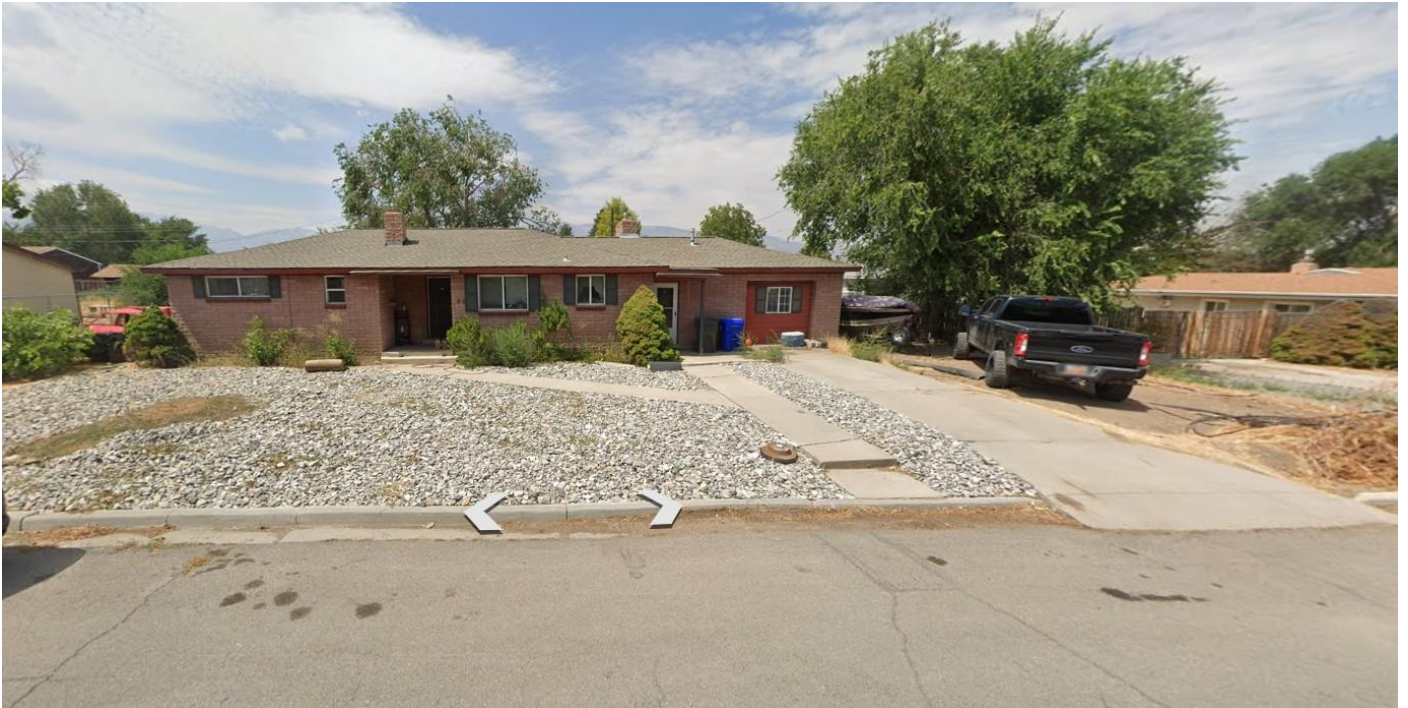
Picture taken 8/2024, prior to the installation of the unauthorized secondary access and before the water meter box was encased in concrete.
