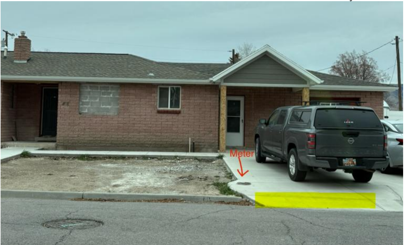
Picture taken 12/31/2025: Yellow box indicates the location of the unauthorized secondary access.
