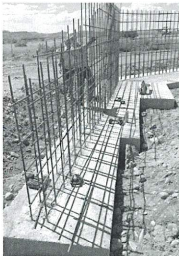
(Construction of Aneth Chapter solid waste transfer station)
