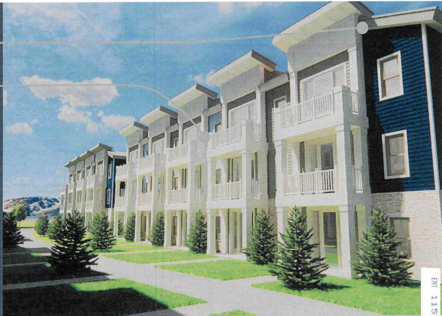
Right front of 5 Unit Townhome Block
