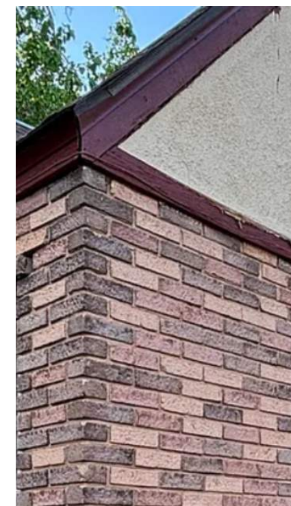
EXISTING BRICK, WOOD MOLDING AND STUCCO TO REMAIN
