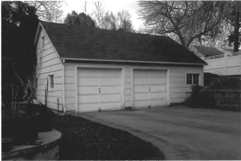
3377 S. Oakwood Street (garage) Photograph 33
