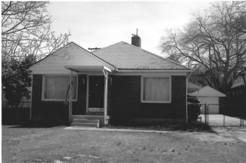
3335 S. Pioneer Street Photograph 35
