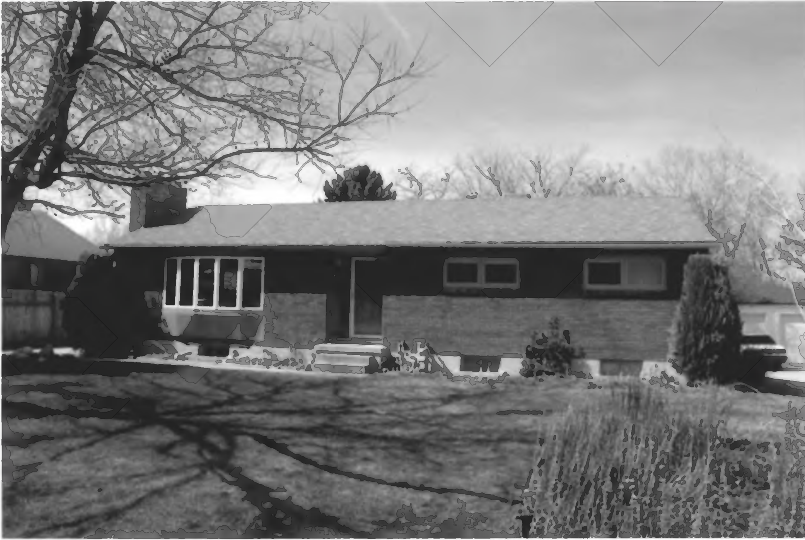
3336 S. Pioneer Street Photograph 41
