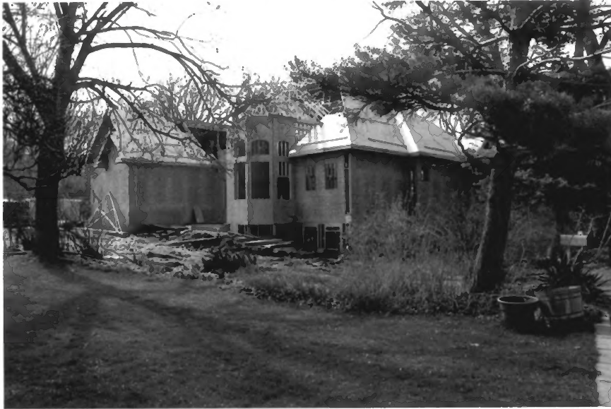
2448 E. Evergreen Avenue (under construction 2006) Photograph 9
