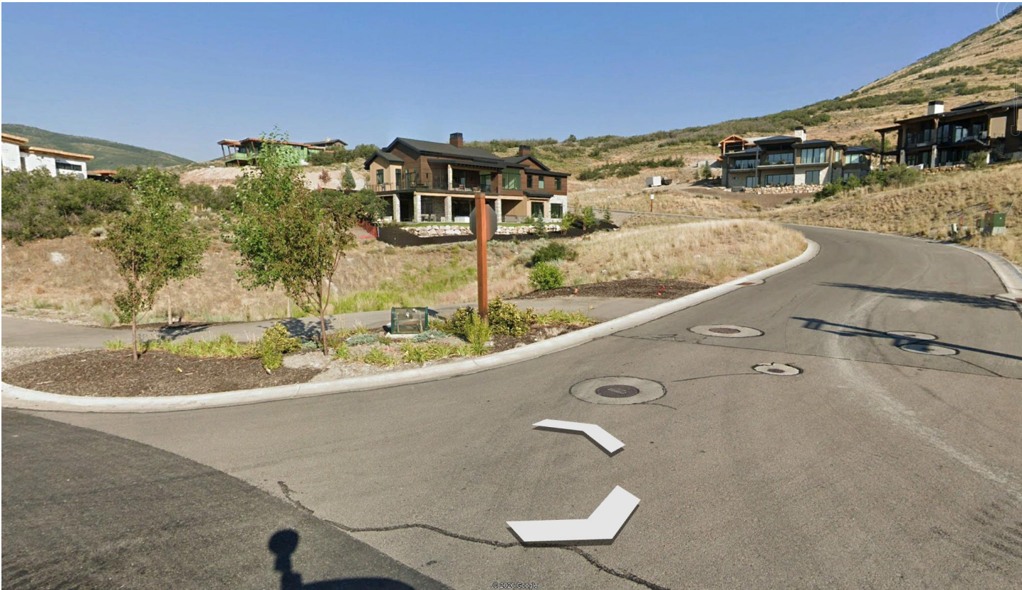
Intersection of Jordanelle Parkway and SkyRidge Drive
