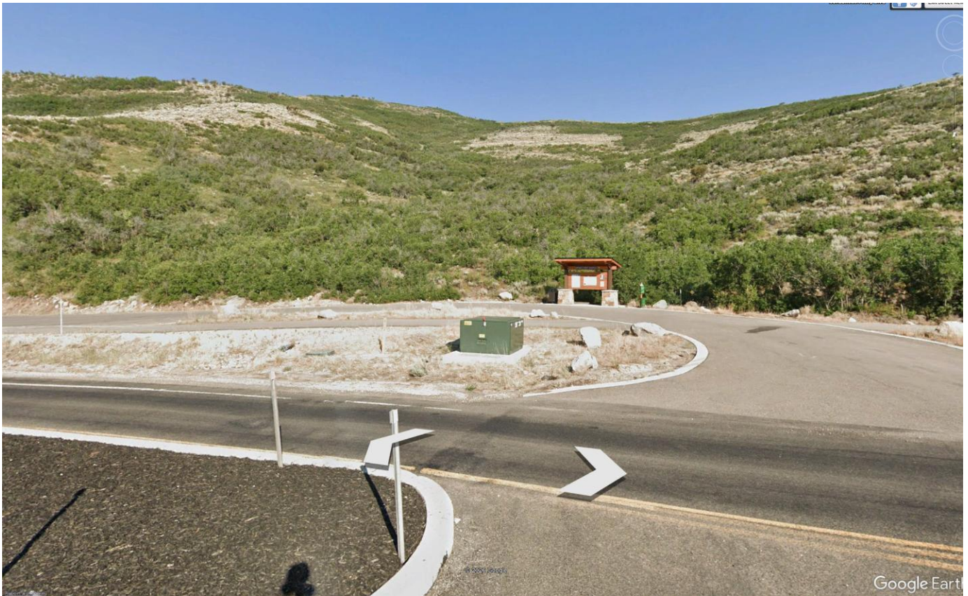
SkyRidge trailhead and Jordanelle Parkway
