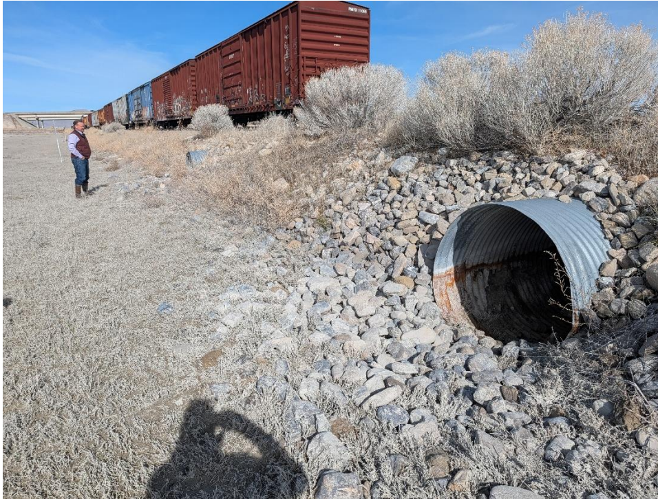
Figure 1-Location of proposed Outfall 001, looking north.
