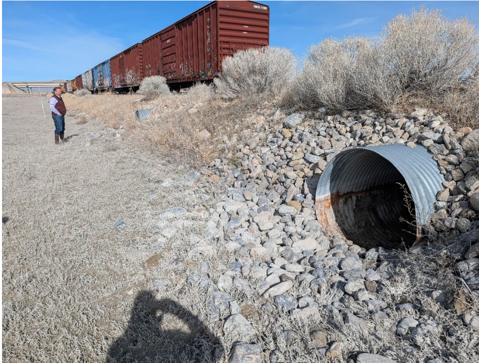
Figure 1-Location of proposed Outfall 001, looking north.
