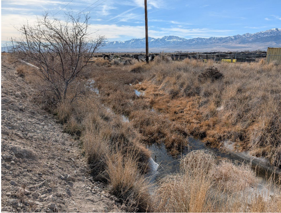
Figure 5-Surface water prior to culvert at Higley Road.
