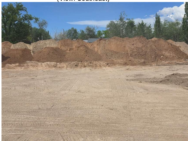
Material Stockpile (View: North)
