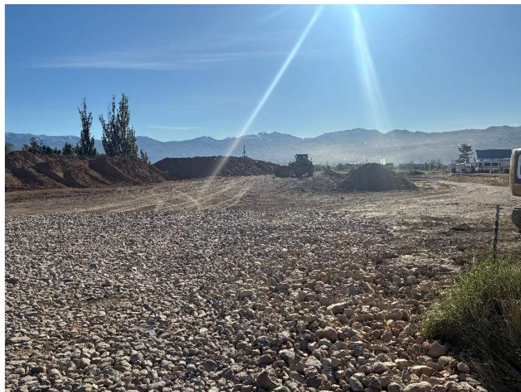
Construction Access (View: Northeast)
