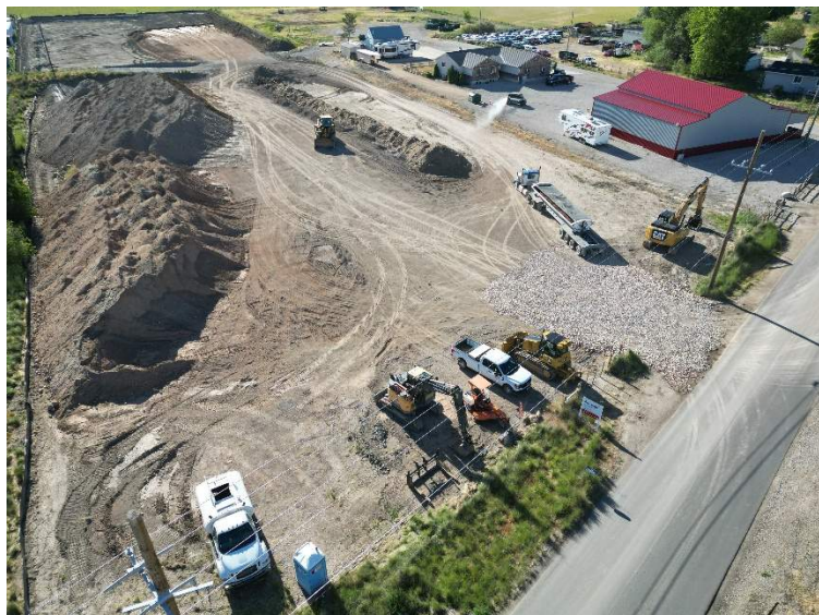
Construction Access (View: Southeast)
