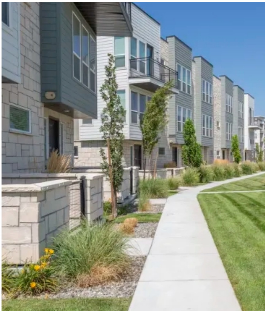
*TOWNHOME PROJECT COMPLETED
