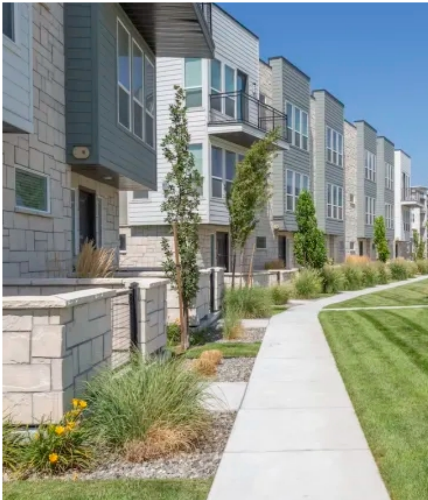
*TOWNHOME PROJECT COMPLETED
