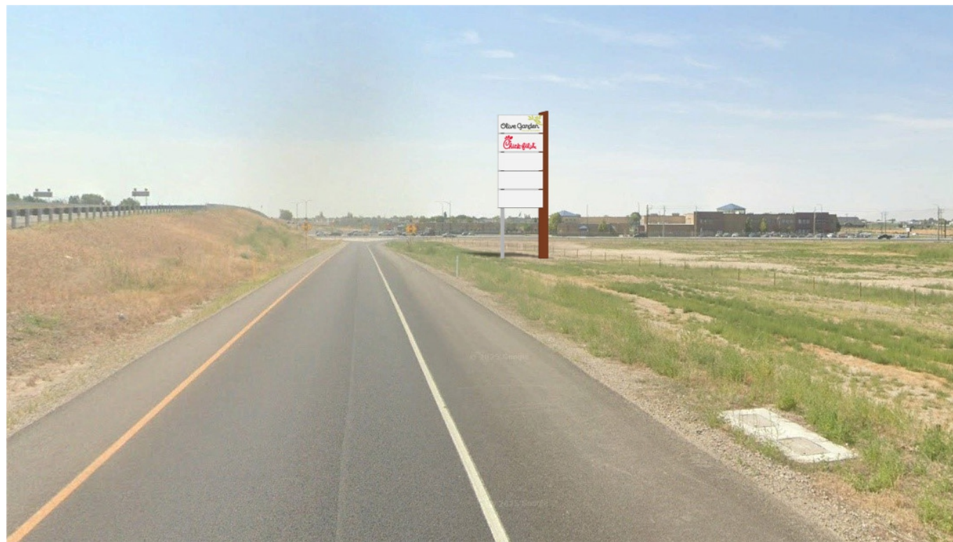
NORTH BOUND 177, EXIT RAMP
