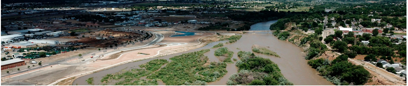
Las Colonias Park Slough Restoration + Boat Ramp | Colorado River, Grand Junction, CO
