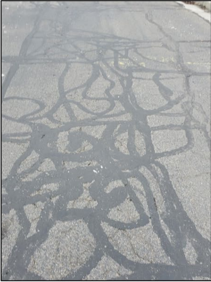
4200 South 3900 West- No cross slope or crown, which results in hazardous ponding at times and ponding in the crosswalk.
