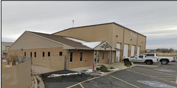
Existing Public Works and Parks Department Building.
