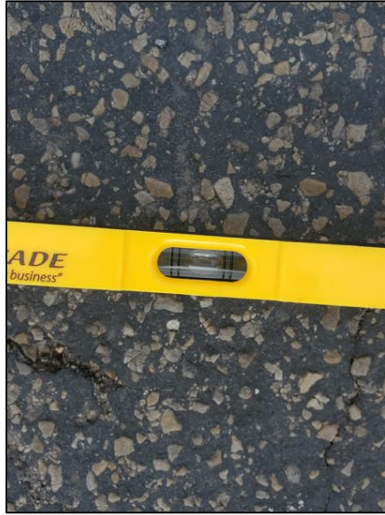
4200 South 3900 West- No cross slope or crown, which results in hazardous ponding at times and ponding in the crosswalk.
