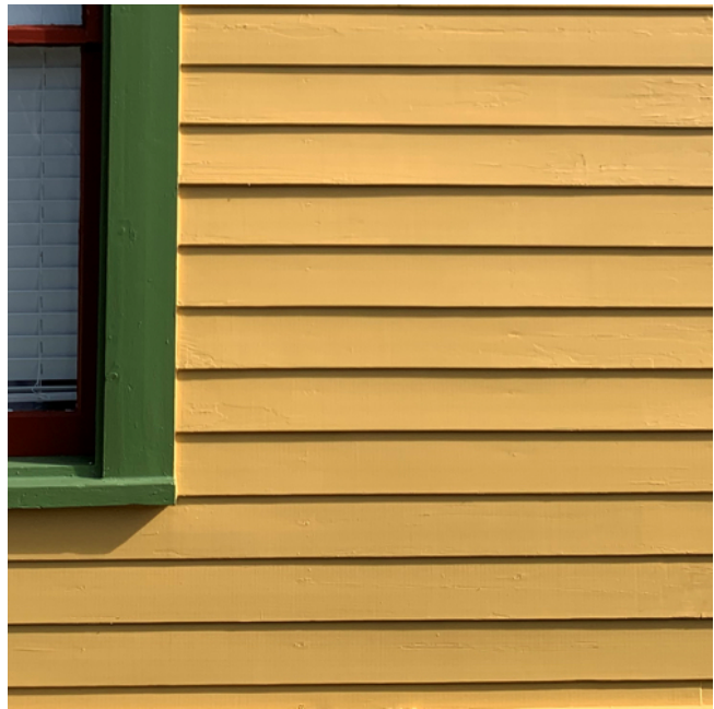
Figure 1: historic profile - lap siding
