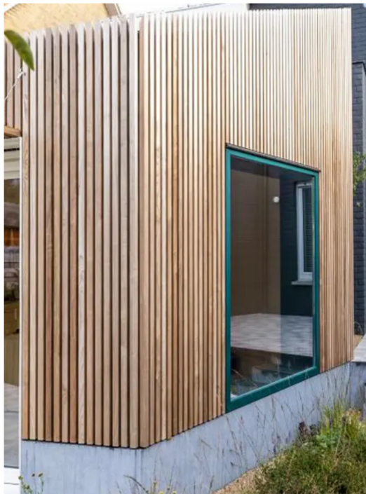
Figure 2: Rainscreen cladding with narrow vertical slats
