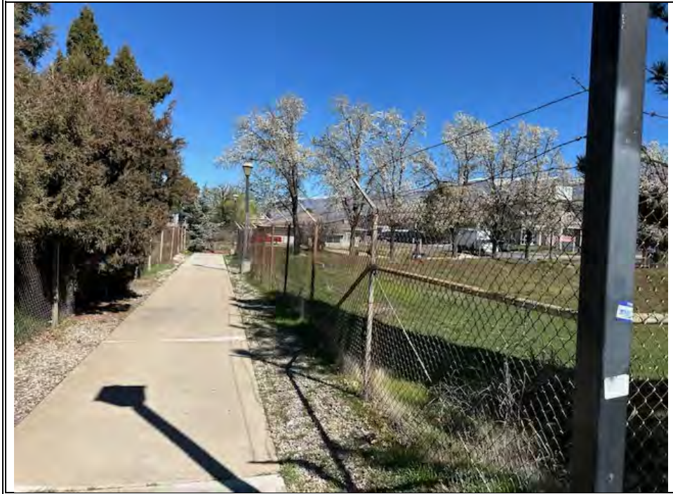
Looking North Along Edge of Detention Basin, Along Partial Fee Acquisition and TCE
