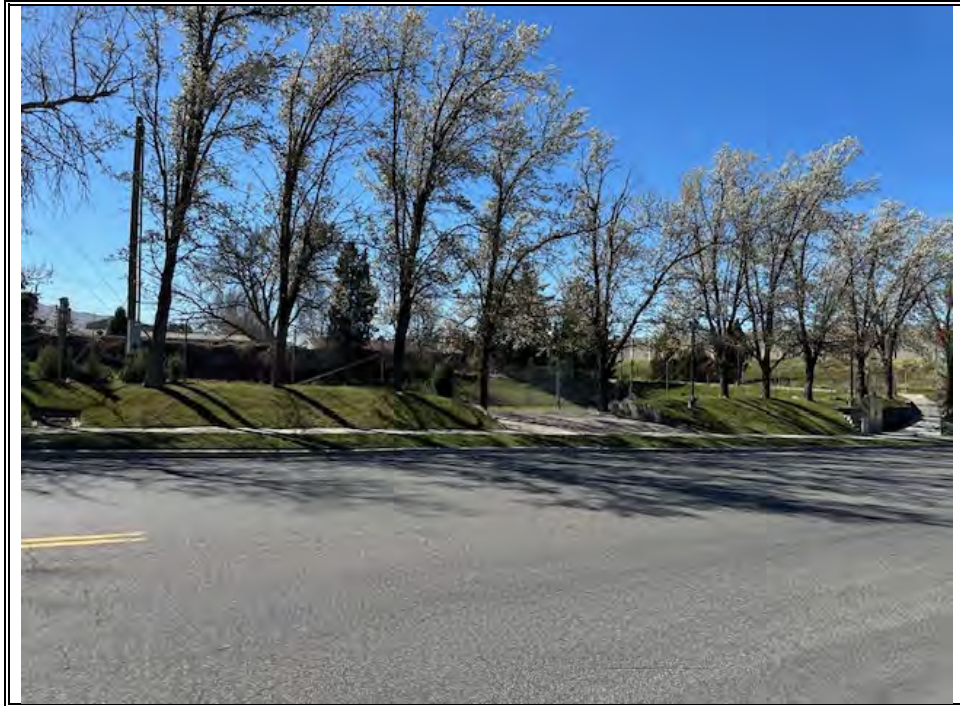
Subject Looking South From 1500 South
