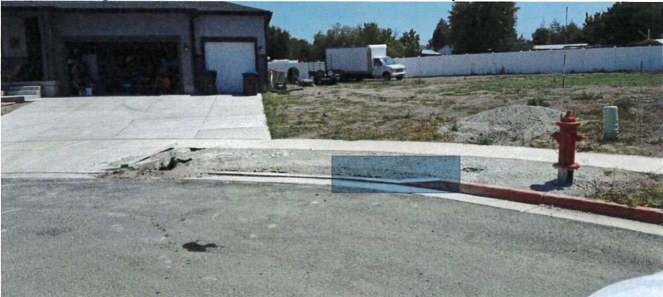
The blue triangle indicates the area where the curb must be replaced
