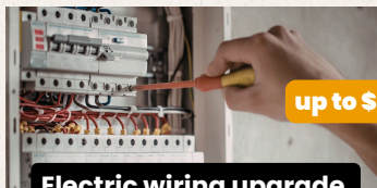
Electric wiring upgrade
