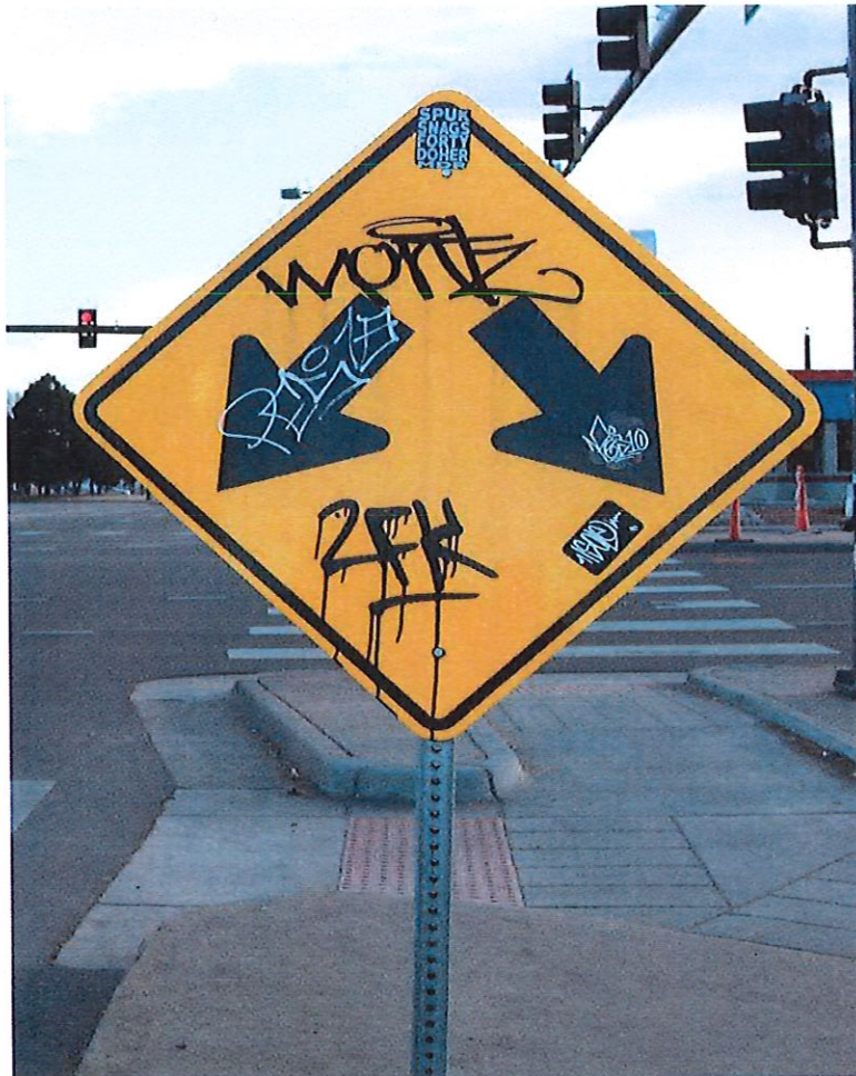
(Shown: Priority 1 - Physical Damage)
