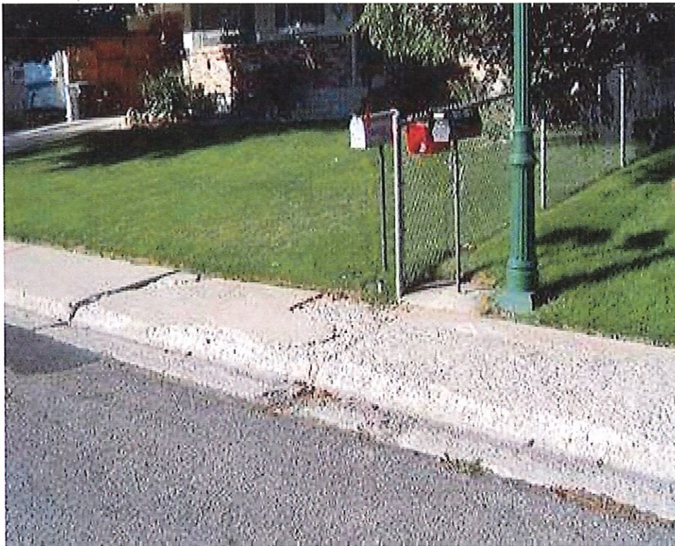
(Priority 1 - Spalling)
