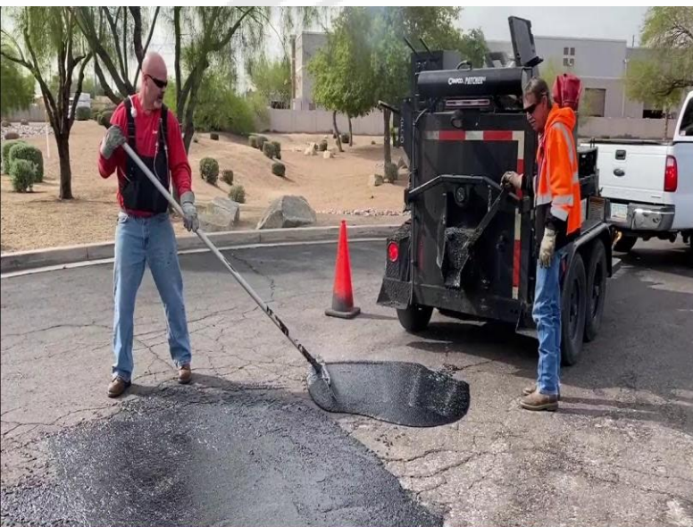
Crafco Patcher II / Mastic One: Skin Patch Repair
