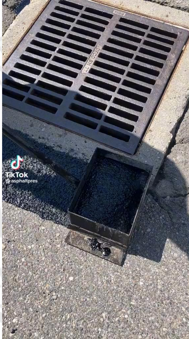
Crafco Patcher II / Mastic One: Skin Patch Repair
