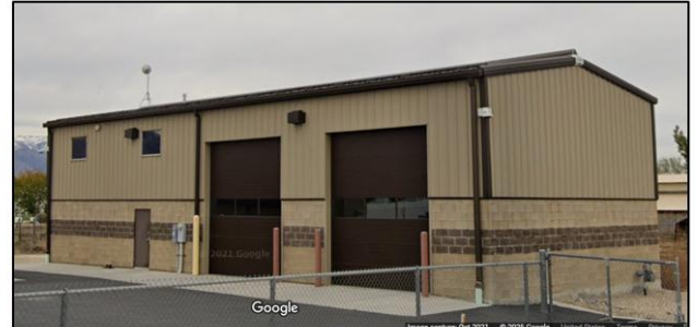
Existing WHHSD Building.
