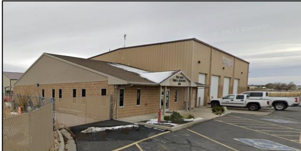
Existing Public Works and Parks Department Building.
