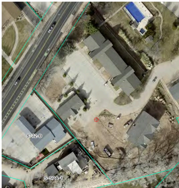
Figure 1. Aerial View showing the area that is currently under construction
