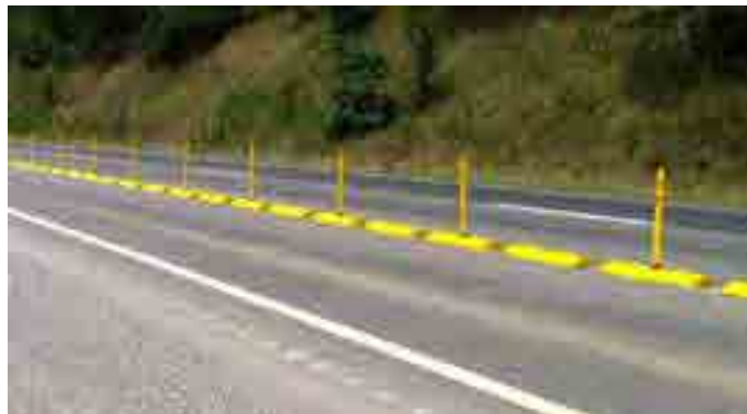
Flexible delineator with rubber curb
