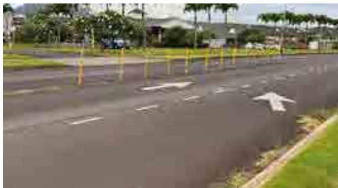
Flexible delineator with rubber curb
