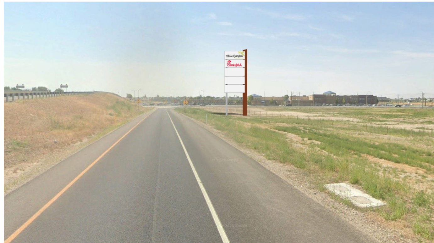
NORTH BOUND 177, EXIT RAMP
