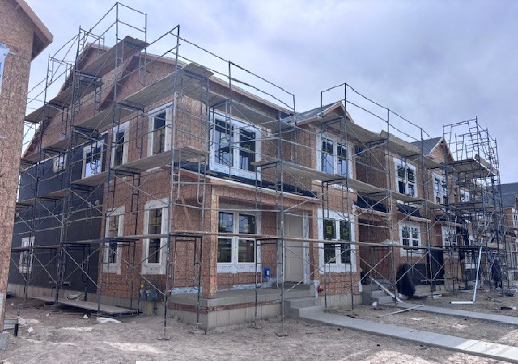
Building 2 (NE corner, from 6200 S)
