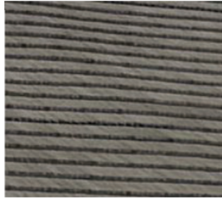
Slate Roofing: existing
