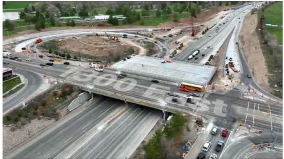
Timelapse of UDOT's I-80 1300 East bridge slide
