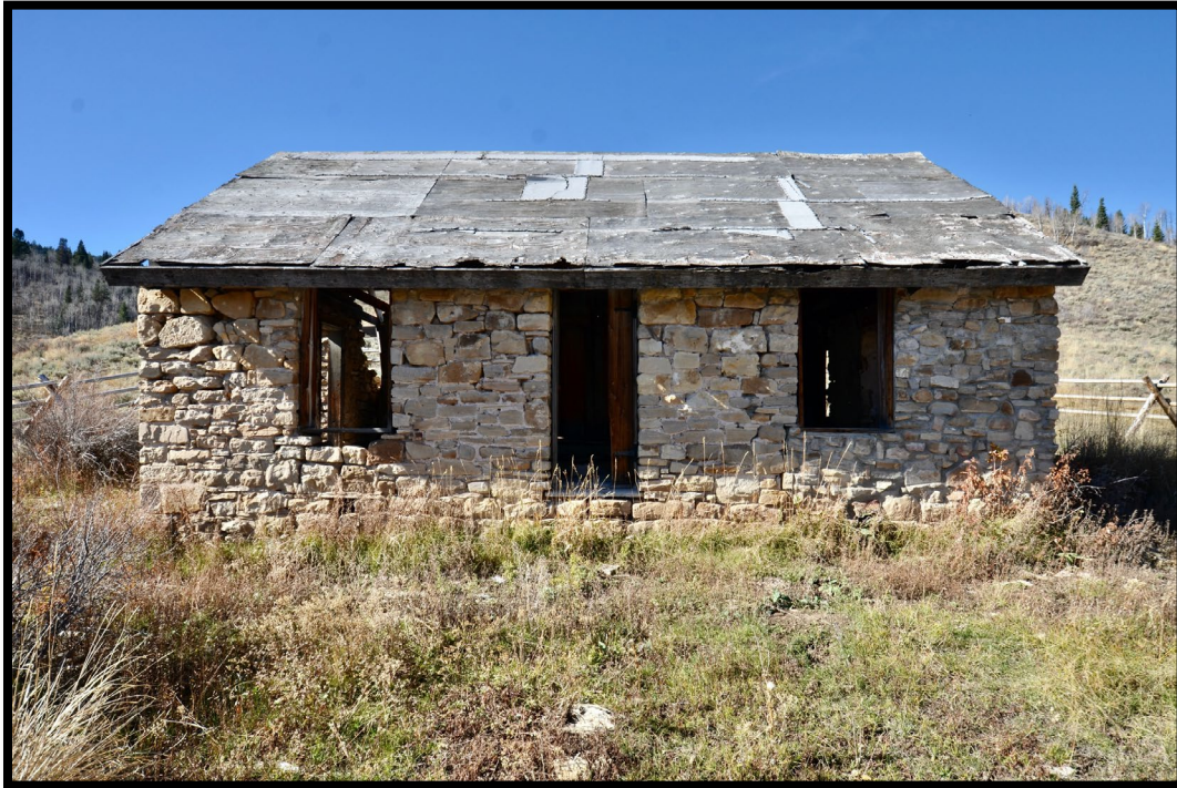
Photo 5: East Façade, View to the West
