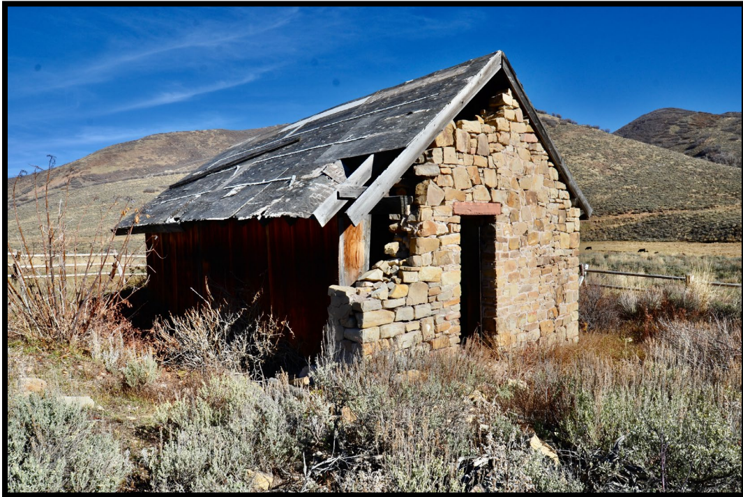
Photo 7: West and South Walls, View to the Northeast
