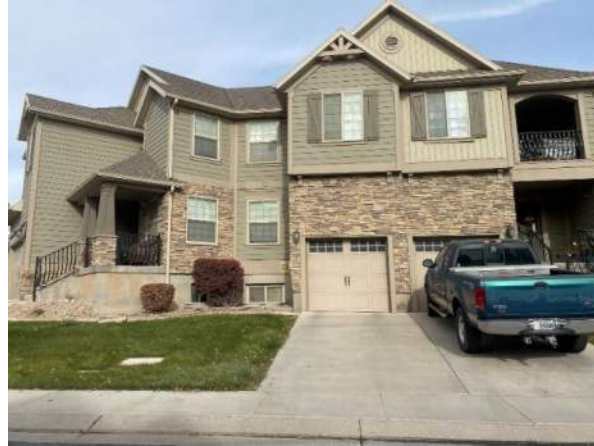
Decorative parapets and multiple roof planes/projections
