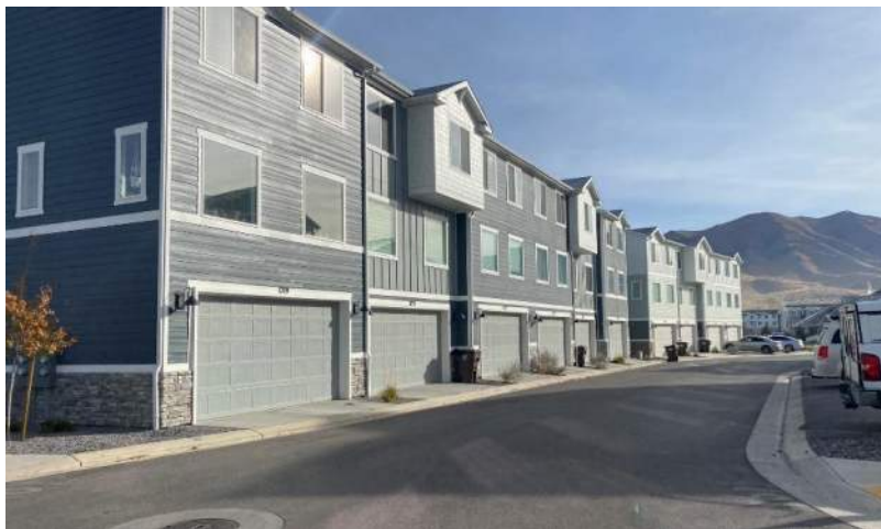
Garages accessed by private service drive
