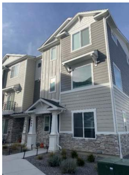
Multifamily unit entry defined with covered porch
