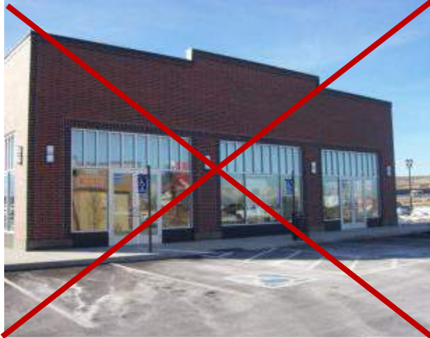
Not Permitted: Entryway not clearly defined; no sheltering element
