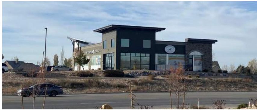
Example of a building located near the front setback, addressing the street with the main entryway visible from the primary street.
