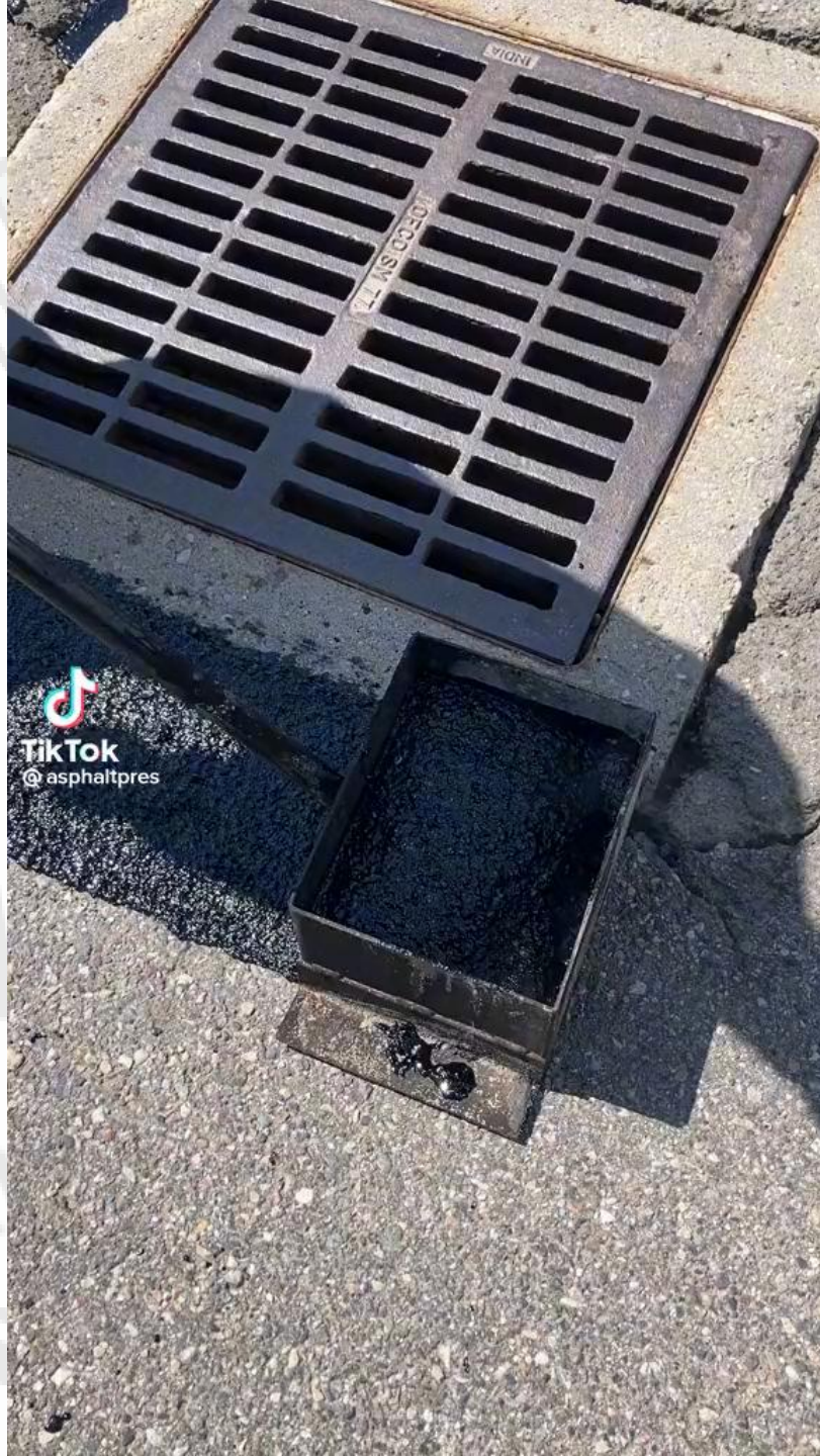
Crafco Patcher II / Mastic One: Skin Patch Repair
