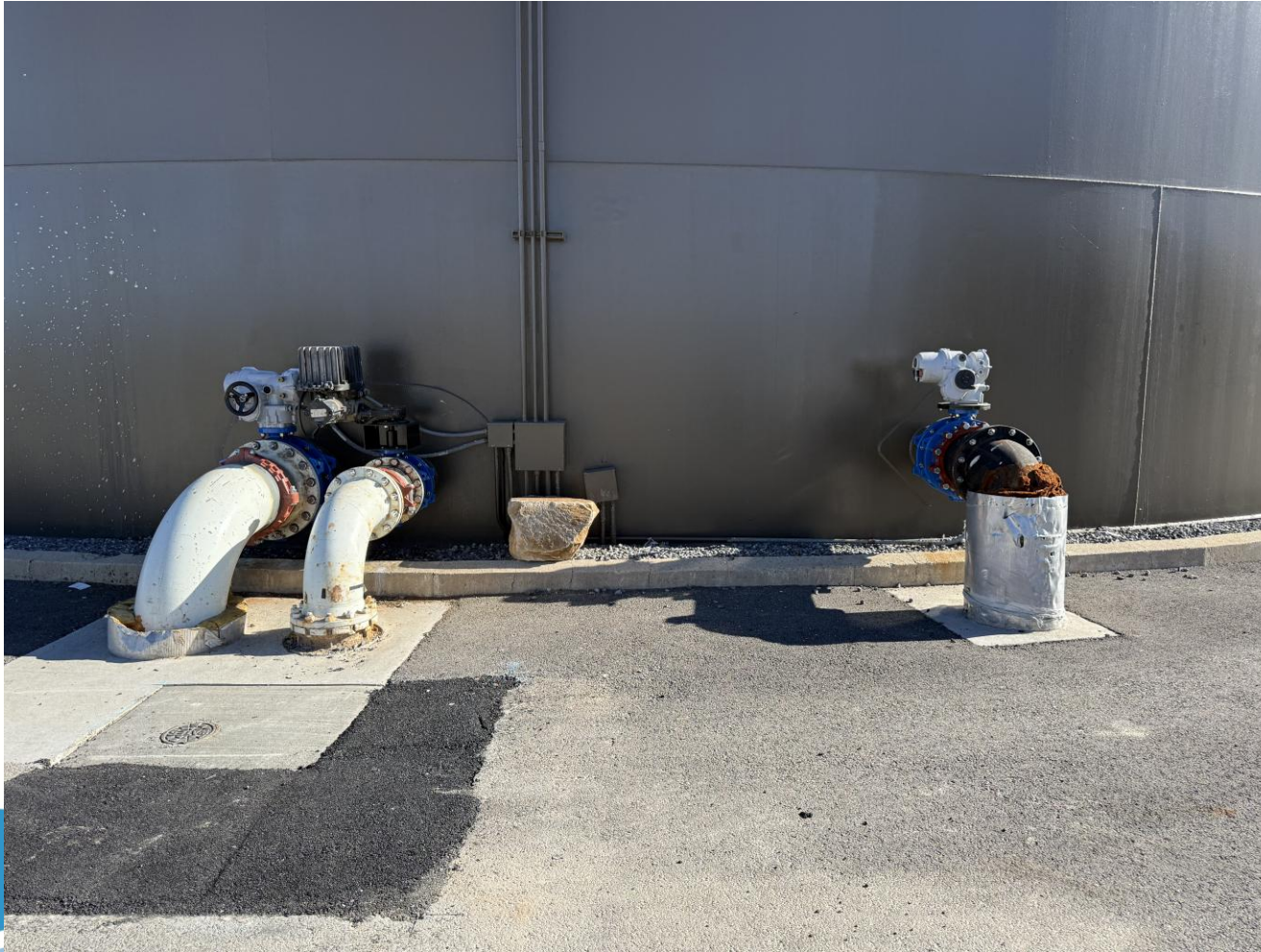
25M Acord Valve & Actuator Replacements
