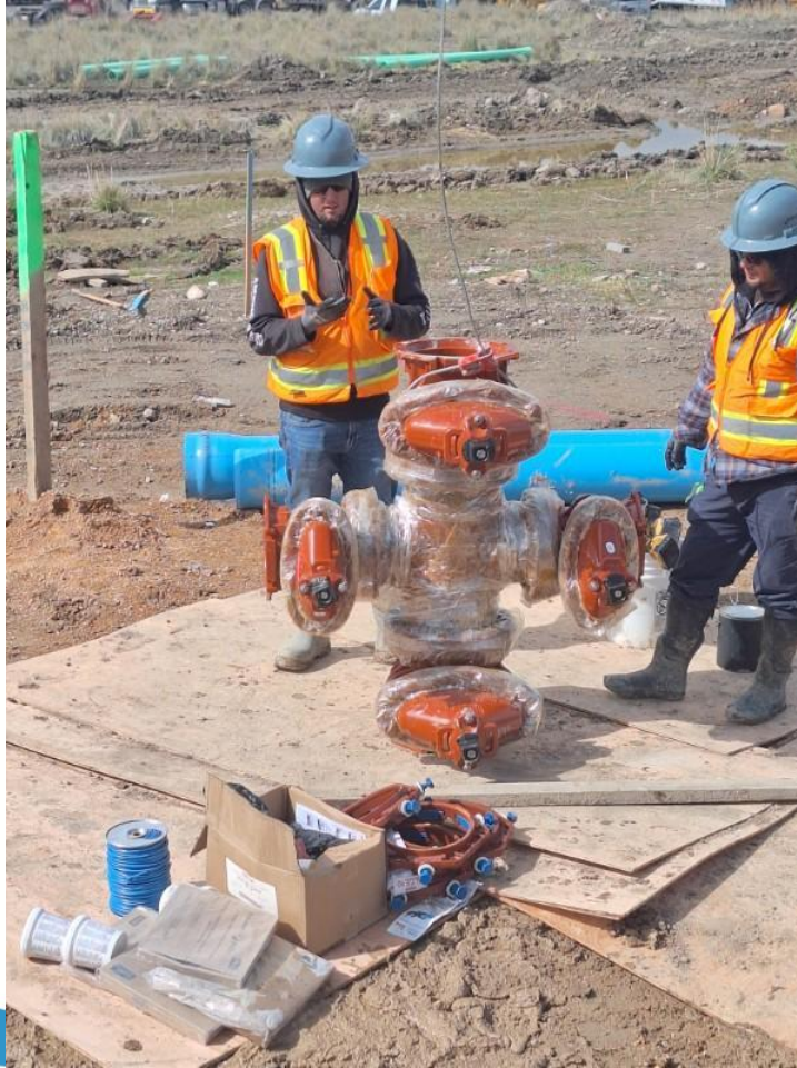
10"x8" tee with valves wrapped with wax tape and poly-ply wrap
