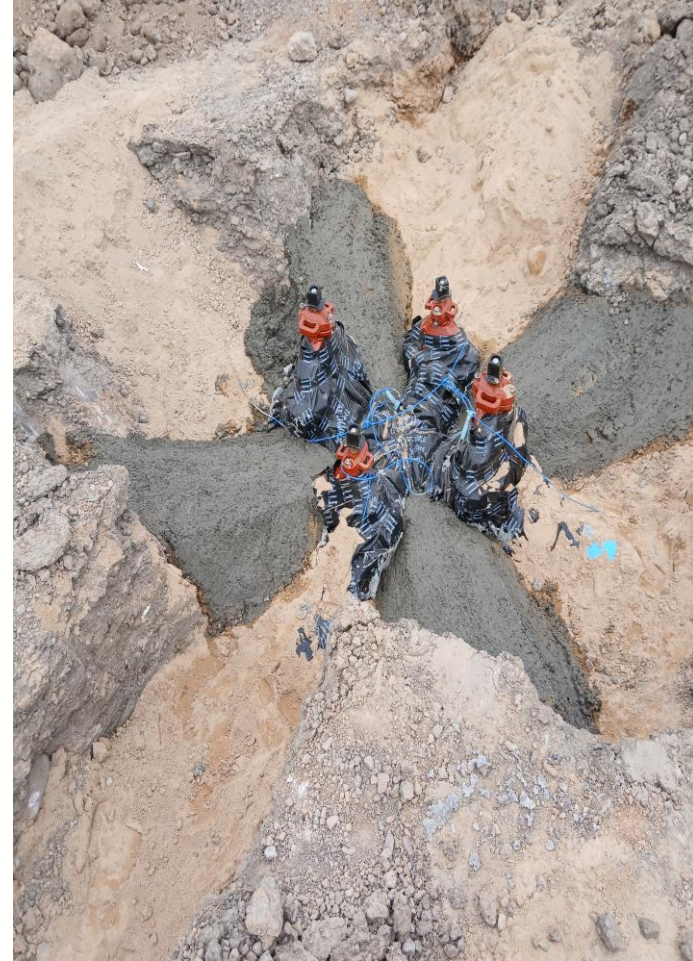
Cross with valves & thrust blocks
