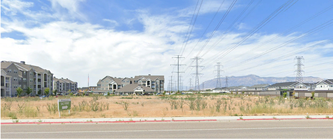
Image 4: Photograph, Existing conditions with RMP Power Lines
