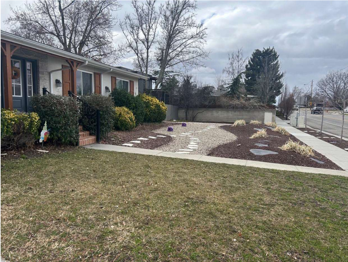
Photo 2 — Front yard overview; there are no sprinklers and we need less depth to pour footings, making this the least disruptive location for construction; neighboring block wall to the right already occupies the visual corridor
