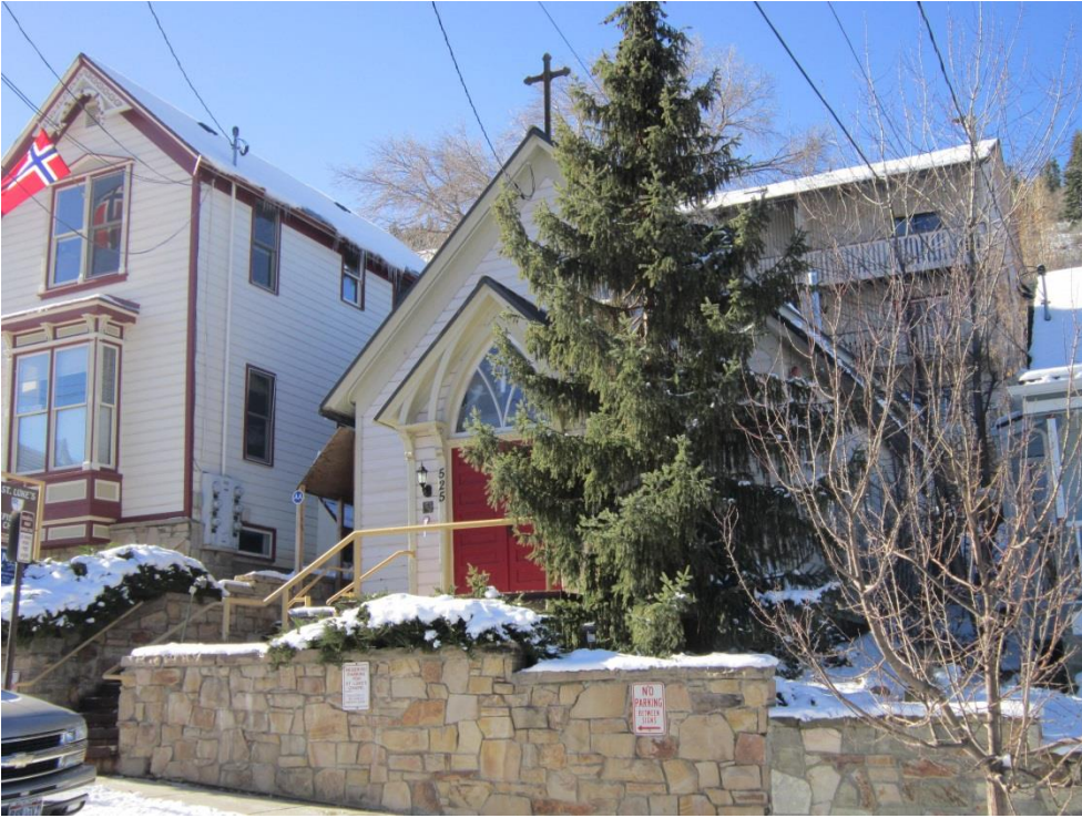
525 Park Avenue. Northeast oblique. November 2013.
