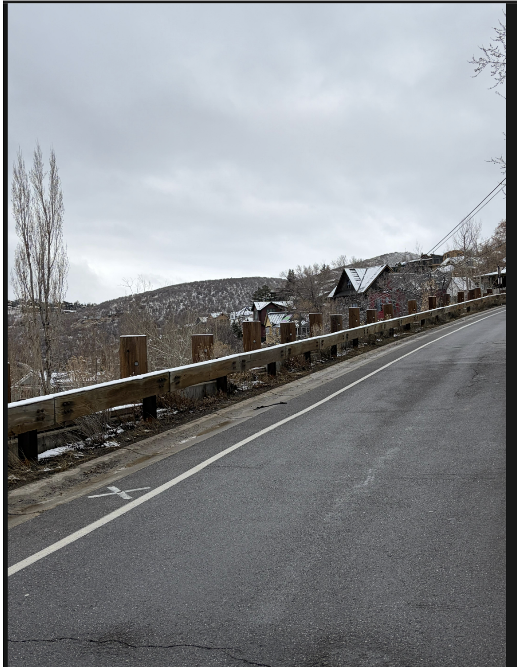
Photo 4. Guardrail/drop-off / constrained edge condition
