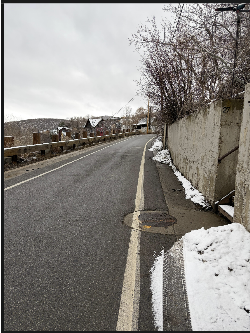
Photo 2. Uphill view from near portal location
