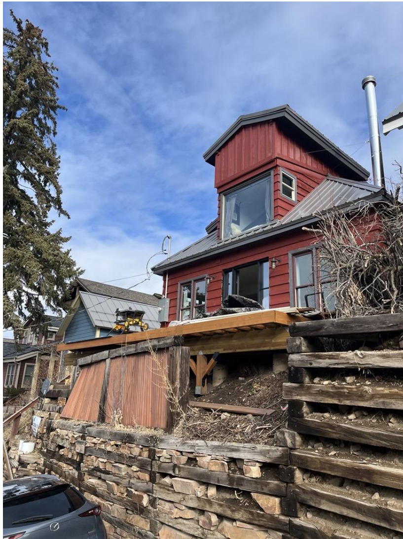
Image 1: New deck under construction at 416 Ontario; photo taken by staff on December 18, 2025.
