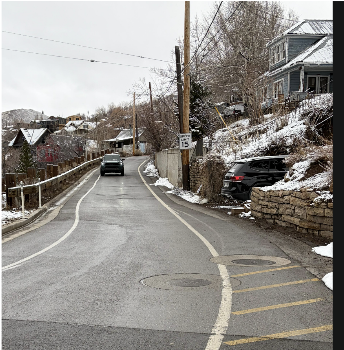
Photo 3. Street edge condition / lack of continuous pedestrian facility
