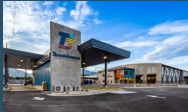
Trans-Jordan Waste Facility
