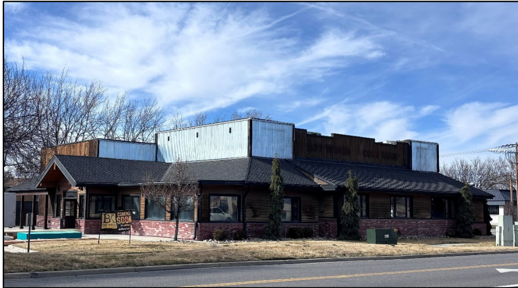
Figure 1 View from 1900 West
