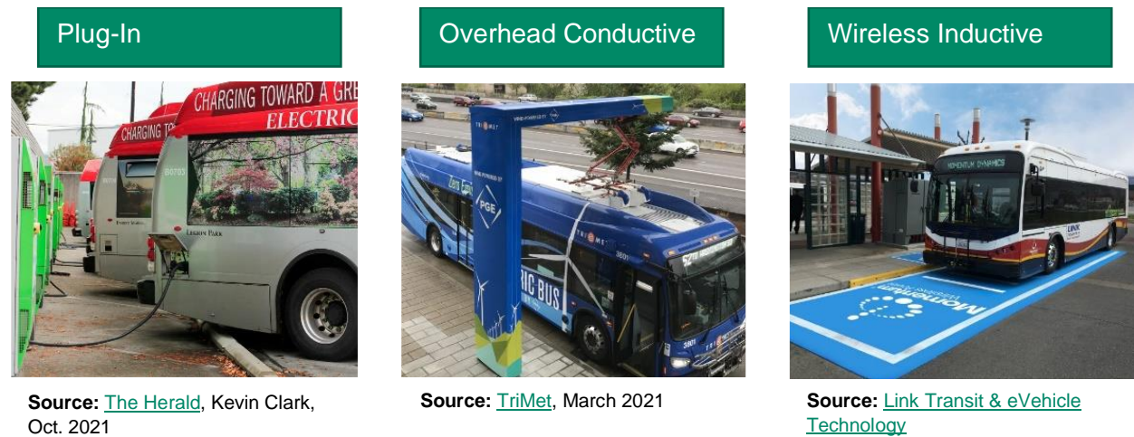
Figure 3: BEB Charging Infrastructure
