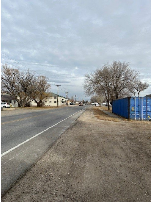
Mid project looking north
