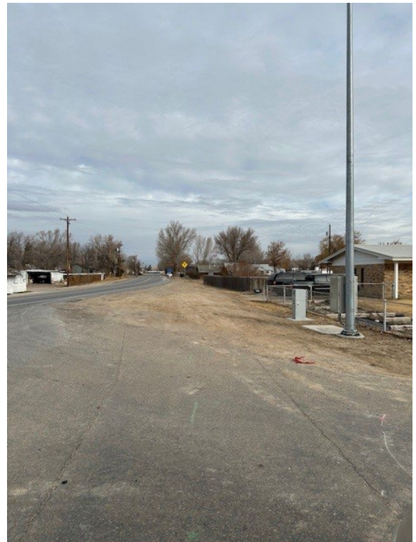
Near end of Project looking north
