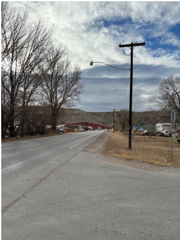
Mid project looking south
