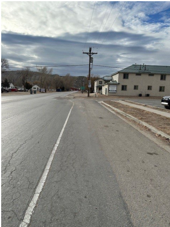
At beginning of project looking south
