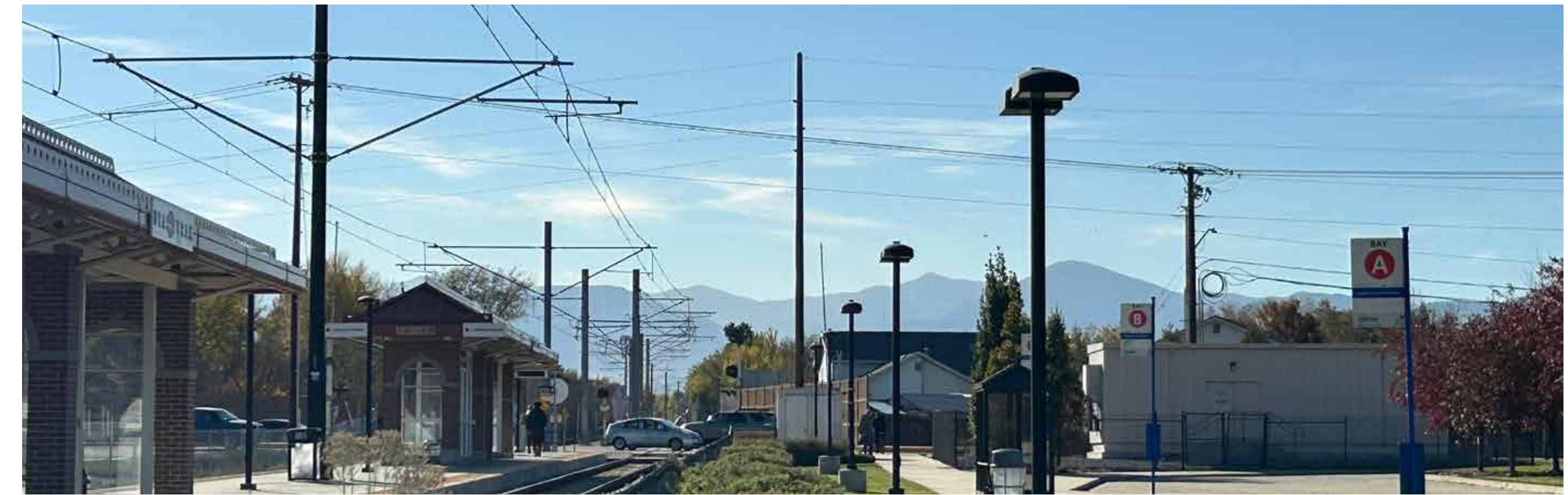
Sugar Factory Road Station Tracks
