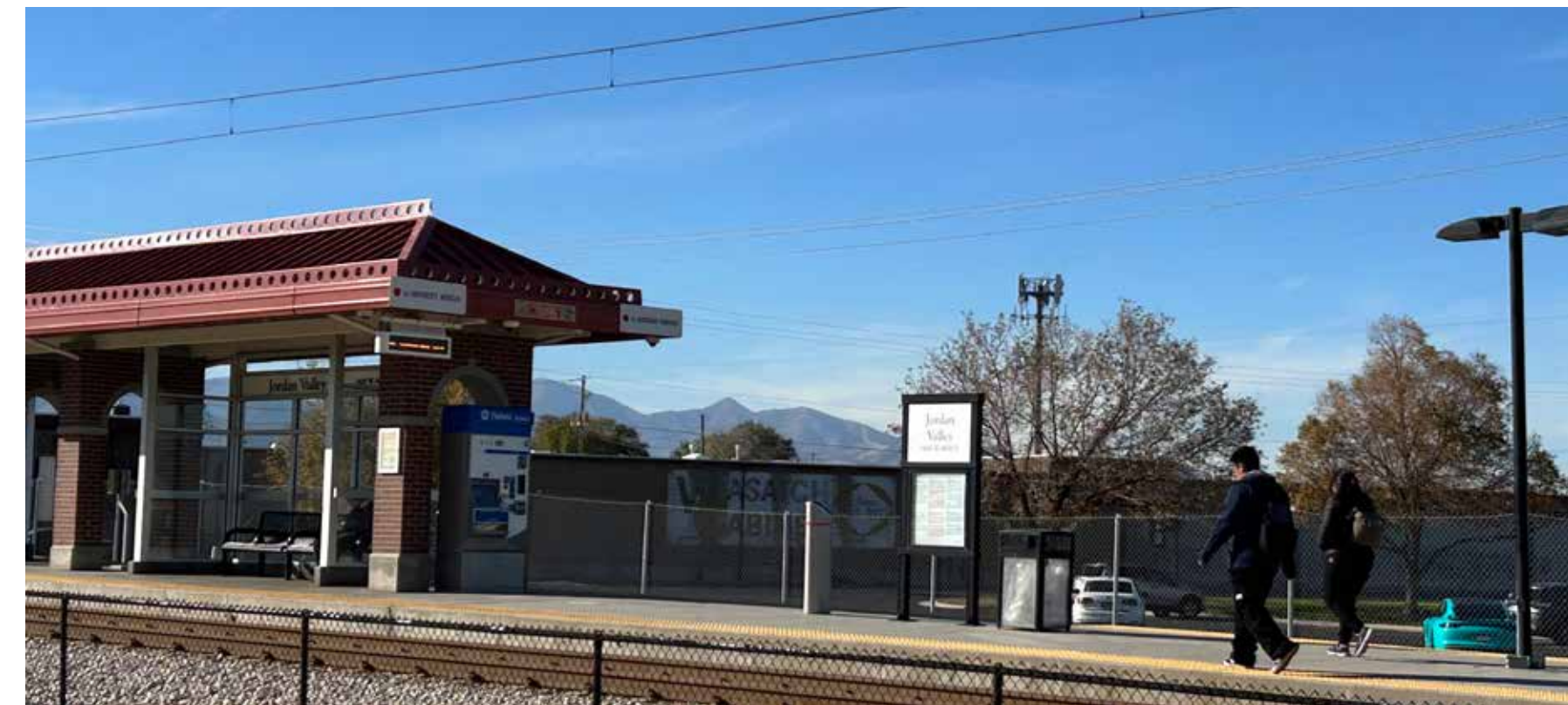
Jordan Valley Station Track
