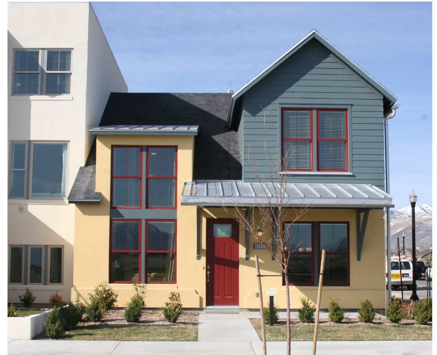
Example of Two Materials (Fiber-cement siding, stucco)
