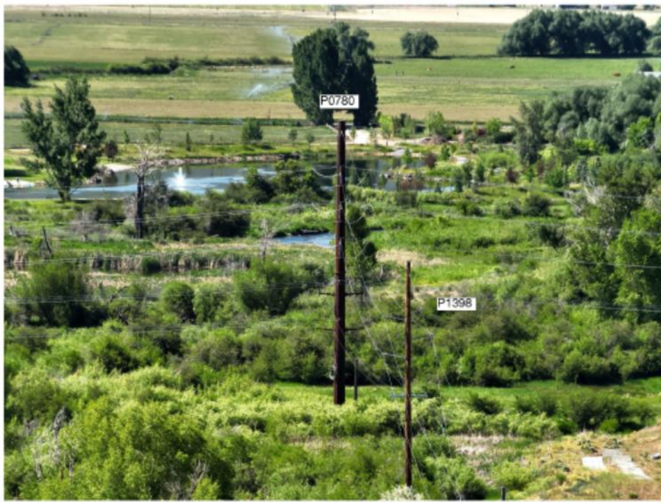
EXISTING POLE(S) - VIEW #1
